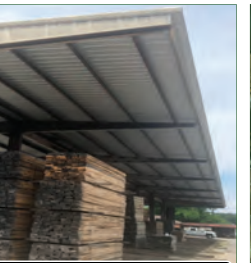
50 ft by 200 ft by 24 ft Prefab metal building (Sell or trade)
