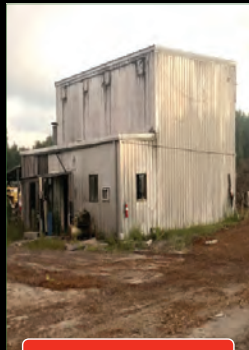
Dry Kilns W/ Motors, Fans, Package Boiler
