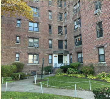
CORONA / NORTHERN BLVD 1 BED, 1 BATH CO-OP WITH FACING FLUSHING SOUND ELEVATED PARKING AND LAUNDRY ON SITE. $125,000
