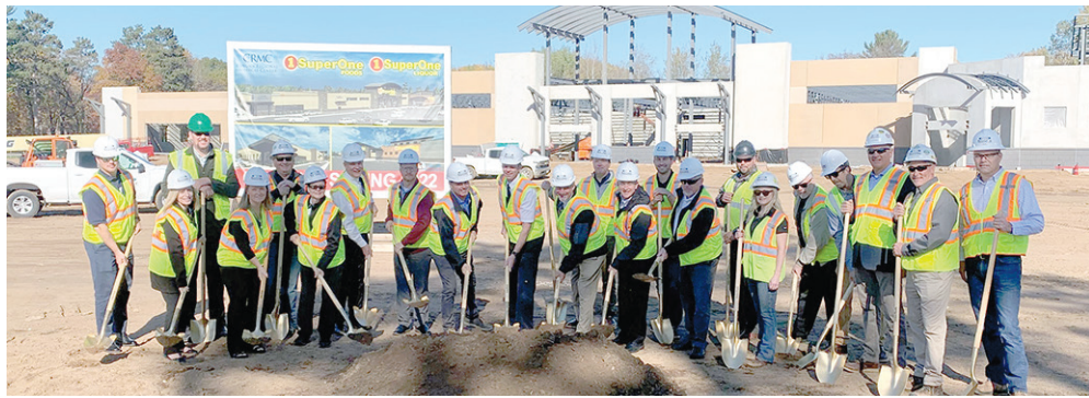
A groundbreaking and progress celebration for Crosby's new Super One Foods, Super One Liquor, and CRMC Clinic was held on Oct 18. The development is at the intersection of Highway 210 and Country Road 31 east of Crosby and is planned for opening the Spring of 2022.
