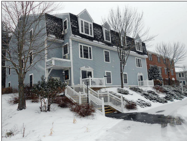
One of the buildings at Schooner Estates had its front yard garden shrubs covered with snow.
