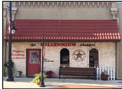
Flippin Printing located inside The Millennium Shopper at 115 Jefferson in Sulphur Springs.
