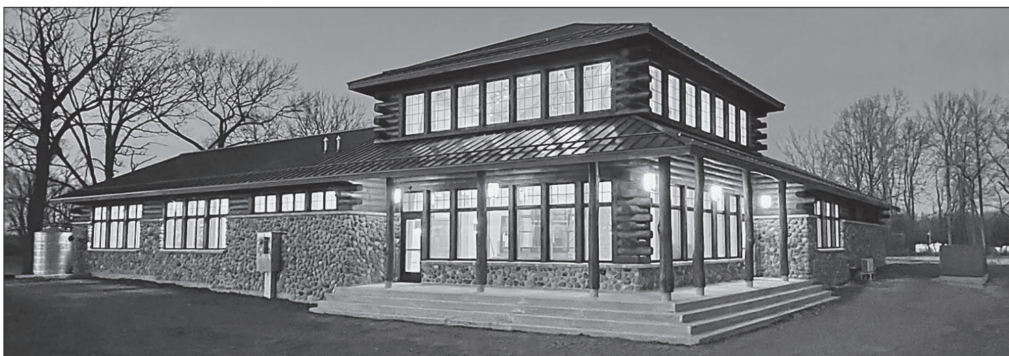
Finishing touches are being put on the new building at the Broughton Sheboygan Marsh. The project is expected to be completed by mid-May.
