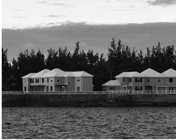
All buildings in Bermuda are colorfully painted in beautiful pastel colors and topped with white roofs.
