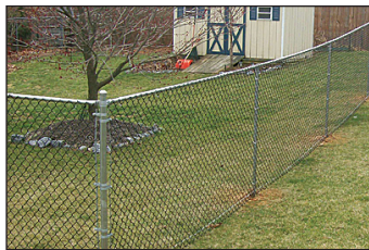
Chain Link Fence
