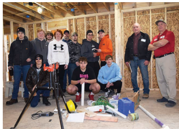
Electrical Class during inspection. Top Row: Alex Montgomery (Newfane), Hunter Bullock (Lockport), Logan Balcom (Medina), Camden Rowles (Newfane), Electricity teacher aide Mark McCabe, Jake Miller (Newfane), Drew Sandolini (Barker), Orion Groth (Albion). Inspector Tim Enderby (Empire Inspections), Teacher Bill Leggett and Bottom Row: Jeff Hain (Royalton-Hartland), Brandon DiNeiri (Royalton-Hartland) and Anthony Volpe (Newfane).
