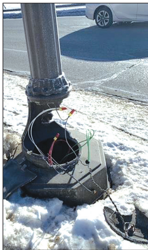
A city light pole damaged by copper wire thieves.
