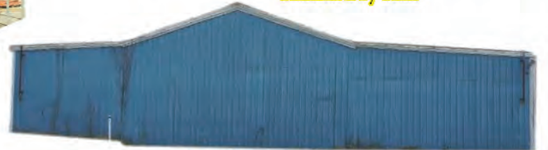
Steel Frame Building
