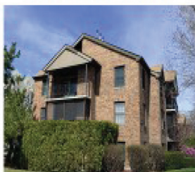
181 Buttrick Avenue, BX 10465 Condo Unit #10B
