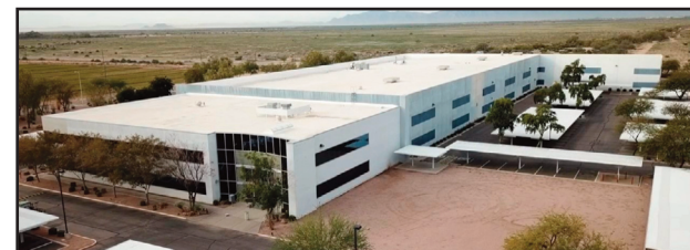
Price Corridor gains another tech-savvy giant, Yield Engineering, and the region gains about 100 jobs at the company's new 123,000 square-foot facility in Chandler.
