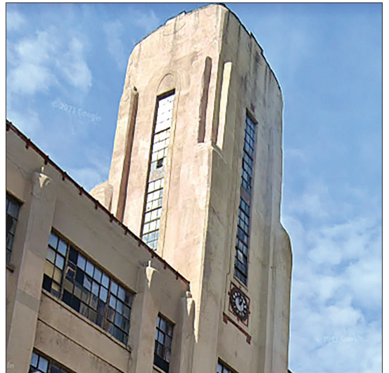
The central tower of the former Saint Paul Casket Company building at 1222 University Ave. The Saint Paul City Council and HRA approved a spending plan on June 22 for converting the nearly century-old building into 55 affordable apartments.
