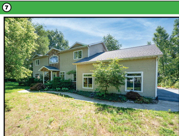
Housing remodel featuring kitchen upgrade Freed Construction Alma - (989) 463-8611
