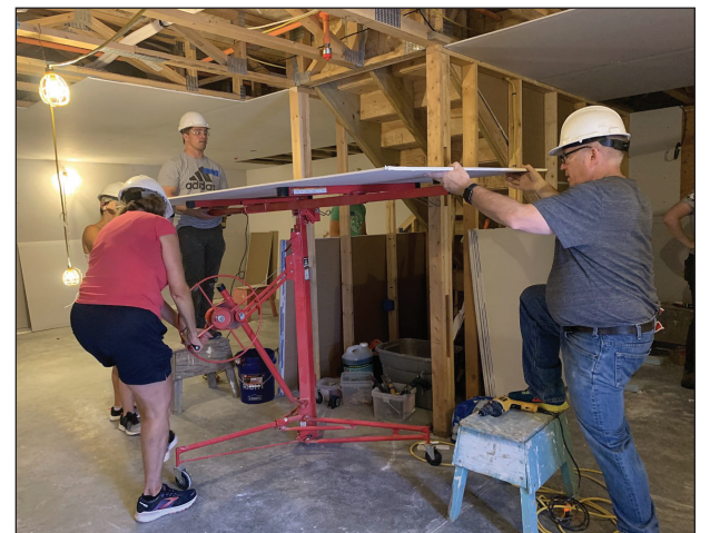
The CMP team sheet rocks the ceiling in the basement.
