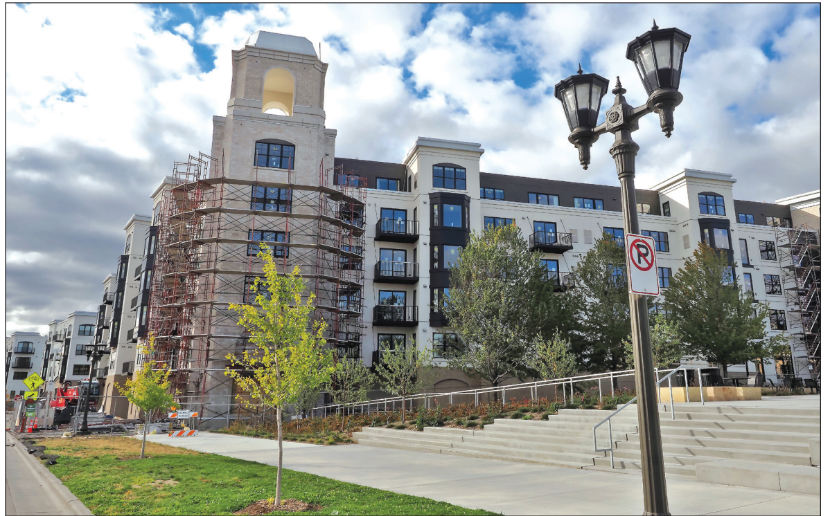
The new Marvella senior housing complex at Highland Bridge is slated to be complete around Thanksgiving and will offer independent living, assisted living and memory care units for those 55 and older. PHOTOS BY BRAD STAUFFER
