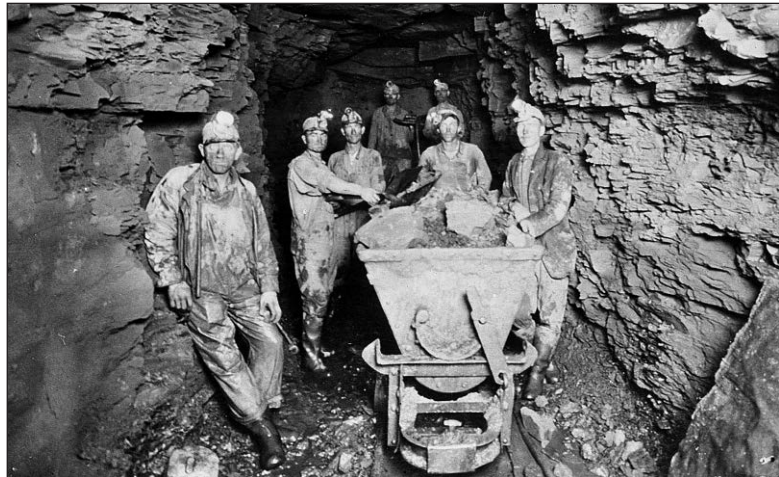
THE TIAWAH TUNNEL: Perhaps the most challenging segment of the 55-mile conduit line was the 84-inch, two-mile-long tunnel bored through the Tiawah hills. This had to be done because the gravity-driven flow of water through the conduit would not have enough "head" to make it over the height of the hills. Thus a large capacity reinforced concrete tunnel through sandstone, shale, coal and clay was constructed.
