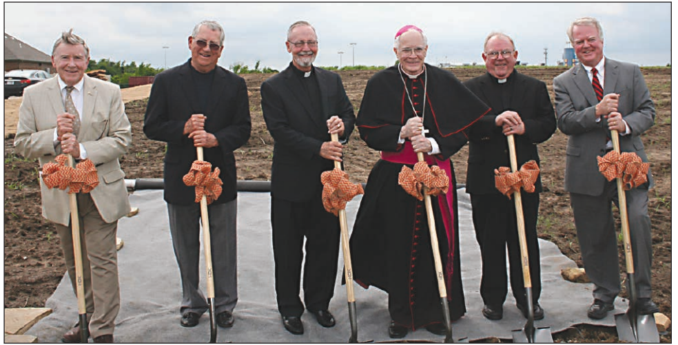
PORTA CAELI GROUNDBREAKING: The groundbreaking for Porta Caeli House was held May 7. From left are Barney Tonquest, Dick Boerger, Msgr. Gregory Gier, Bishop Edward Slattery, Msgr. Dennis Dorney, Bob Sullivan (all are PCH Board members except Dick Boerger, who is a PCH Project Team member). Porta Caeli House is a nonprofit that will be a home for those approaching the ends of their lives. It will be located adjacent to Catholic Charities on North Harvard Avenue in Tulsa.
