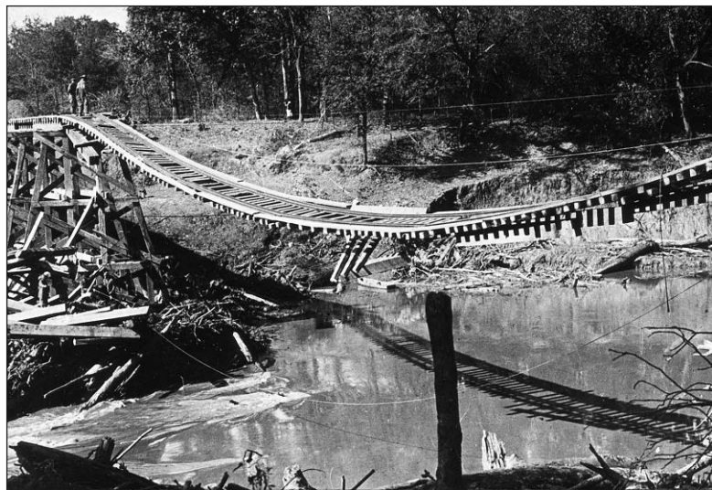
AND THE RAINS CAME: Spring rains stopped work on the Spavinaw waterline at least twice, setting back progress and raising costs.
