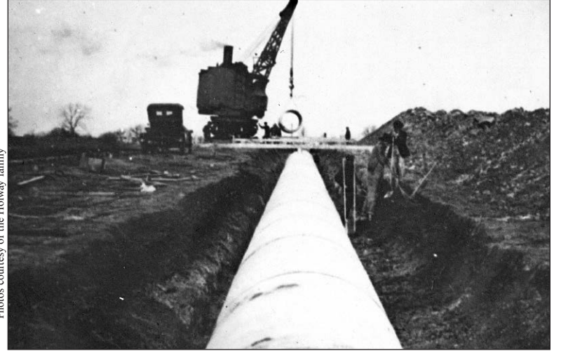
DOWN SHE GOES: It took a 24-ton locomotive crane to carefully lower the ten ton pipe sections into the trench or "cut" as it was called, to join the growing conduit string.
