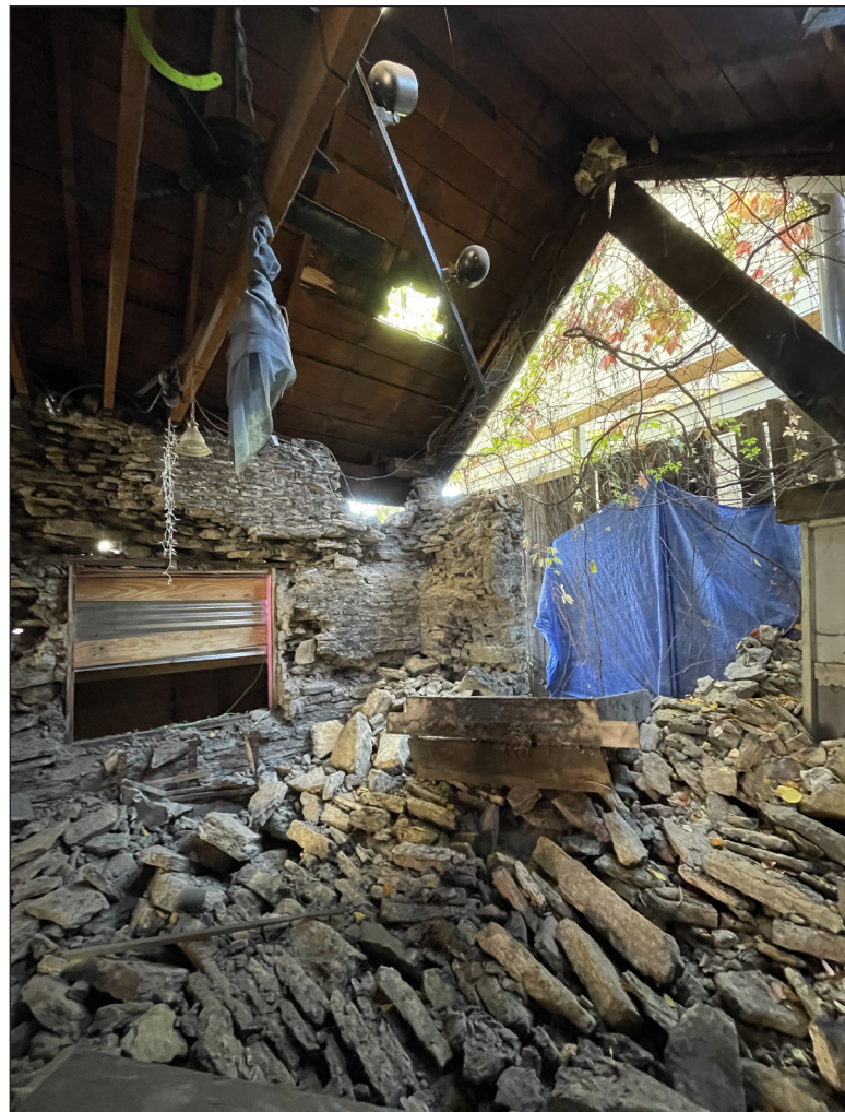
Located on the patio at Burger Moe's restaurant on West Seventh Street, the 170-year-old Justus Ramsey House is looking worse for wear these days. The roof has a gaping hole, and a wall has collapsed into the interior (right).
