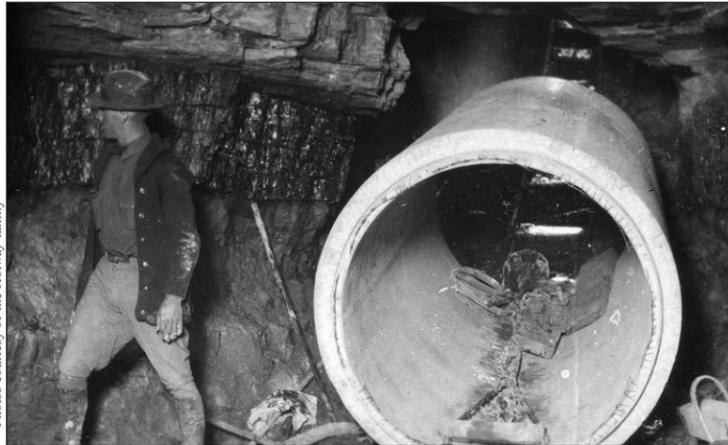
**THE VERDIGRIS TUNNEL:** The Verdigris tunnel required a subterranean excavation seven hundred feet long primarily through solid limestone creating a cave seven feet in diameter, large enough for the 54-inch conduit pipe to be laid and encased in grout.
