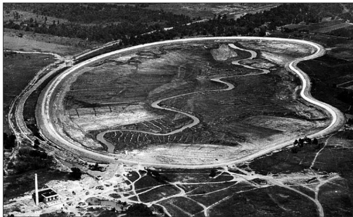
**BRING IT ON:** The site for the Mohawk reservoir shown here under construction in mid 1923 was chosen because of its above sea level elevation being a mere 75 feet below the top of the soon to be completed Spavinaw dam spillway. Holway persistently proclaimed there was enough drop to provide adequate head for the proposed gravity flow waterline. He did so in the face of stiff opposition from many doubters.
