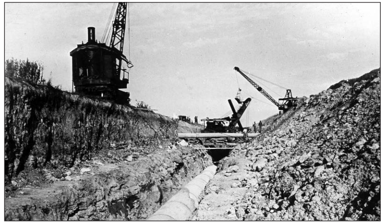
THE CUT: The trench, or cut, sometimes went as deep as 40 feet. Pictured here is a more common cut of approximately 25 feet. The top half being prairie soil, the bottom half pesky shale presented challenging excavation.
