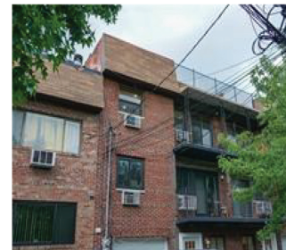
276 Buttrick Avenue I3, BX 10465
