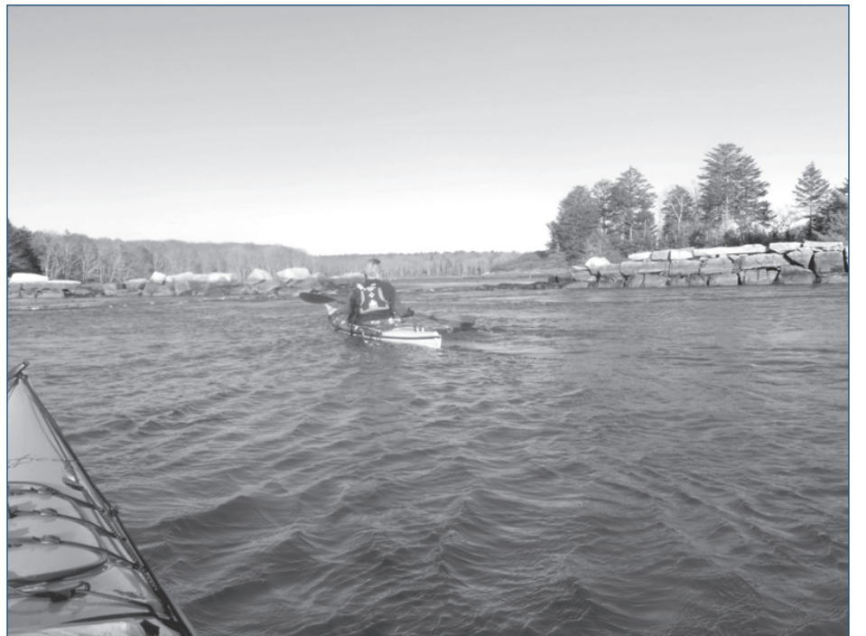
Remnants of a washed out dam are encountered at the outlet of Spirit Pond
