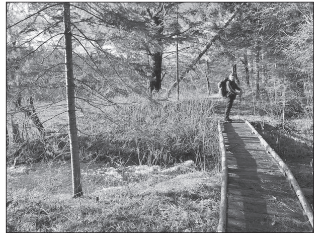
One of several wooden bridges on Seboeis Riverside Trail
