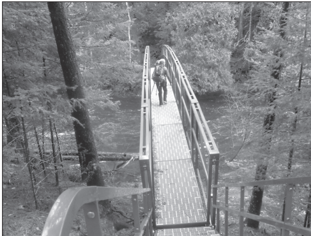
An impressive metal bridge has been built high over Shin Brook
