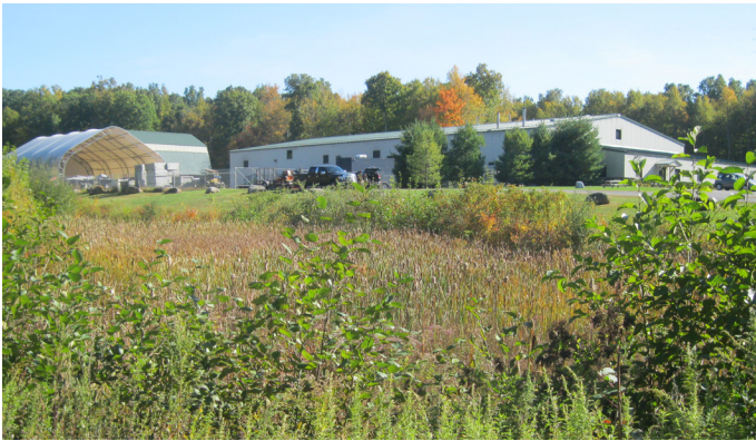
Coventry DPW garage and case study drainage: A view of the DPW garage in the background. In the foreground is one of the property's drainage ponds, shaped for proper drainage and planted with native vegetation like cattails. Invasive plants like Phragmites have been removed.
