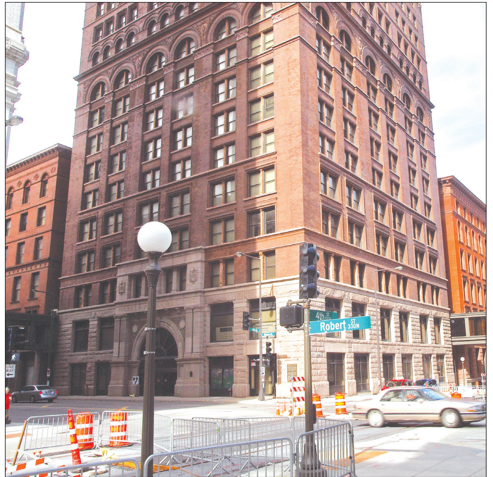
The Pioneer Endicott Building at 141 E. Fourth St. is the first in Saint Paul to receive a conditional use permit for more than four short-term rental units. It's planning to have nine. PHOTO BY BRAD STAUFFER
