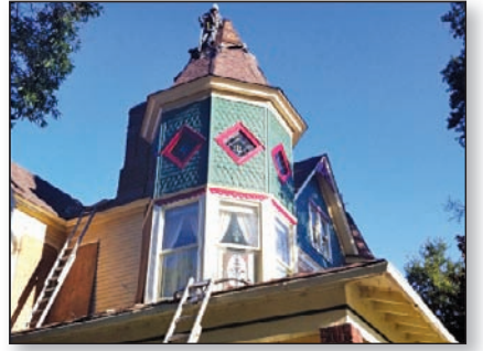
Roofing work is one of WPI's specialties. ChooseWPI.com
