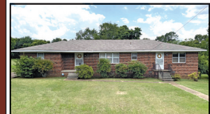
Commercial Potential - 675 Cox Creek Pkwy
