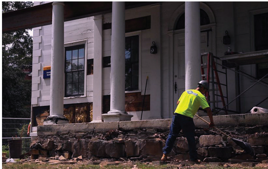
Water damage necessitated the removal of the stone steps leading up to the front door.
