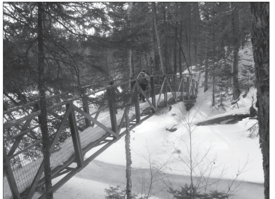
An impressive metal suspension bridge spans Shin Brook on Seboeis Riverside Trail
