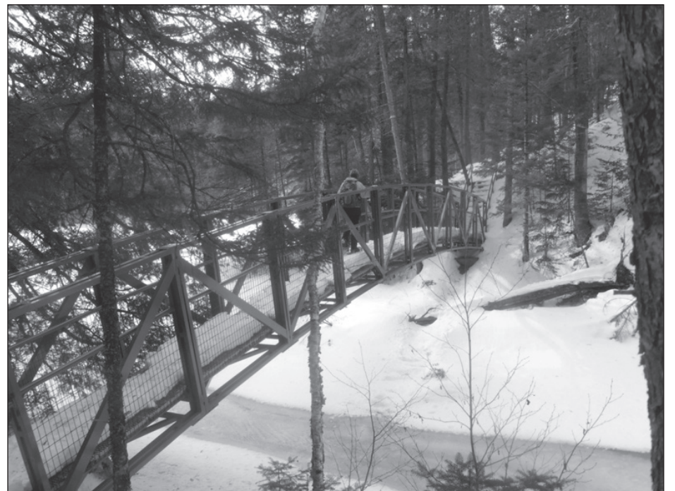
An impressive metal suspension bridge spans Shin Brook on Seboeis Riverside Trail
