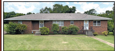
Commercial Potential - 675 Cox Creek Pkwy
