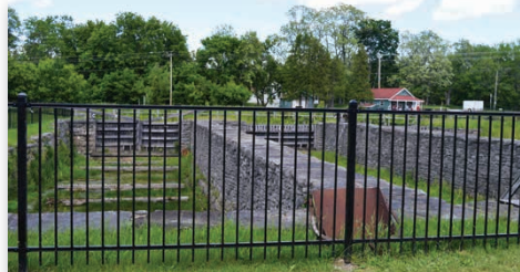
Remnants of dry docks unearthed and restored at the Canal Boat Museum. The dry docks were used to repair canal boats in the early days of the Erie Canal
