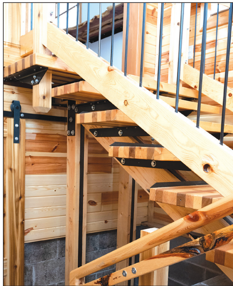
Floating staircases provide access to the home’s main level and basement.
