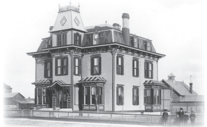
Bresnahan House Photo Courtesy of Wyoming State Archives
