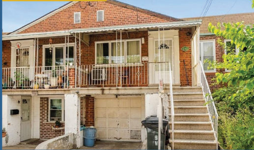
Throggs Neck all brick ranch with 3 room walkout basement. Priced to Sell! Vincent Buccieri, Lic. Assoc. RE Broker 917.440.2122
