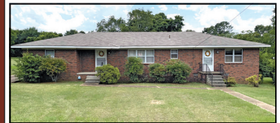
Commercial Potential - 675 Cox Creek Pkwy
