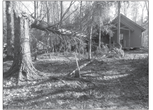
Snowshoe Lodge was damaged by a fallen tree but still habitable
