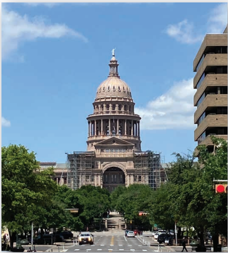
The Texas State Capital building in Austin is a stunning example of architecture that can be seen from quite a distance.
