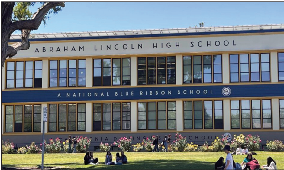
Lincoln High School in San Jose. Photo by Lorraine Gabbert.
