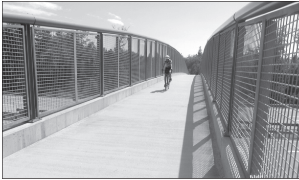
A cyclist traverses Eastern Trail Bridge over Interstate 95
