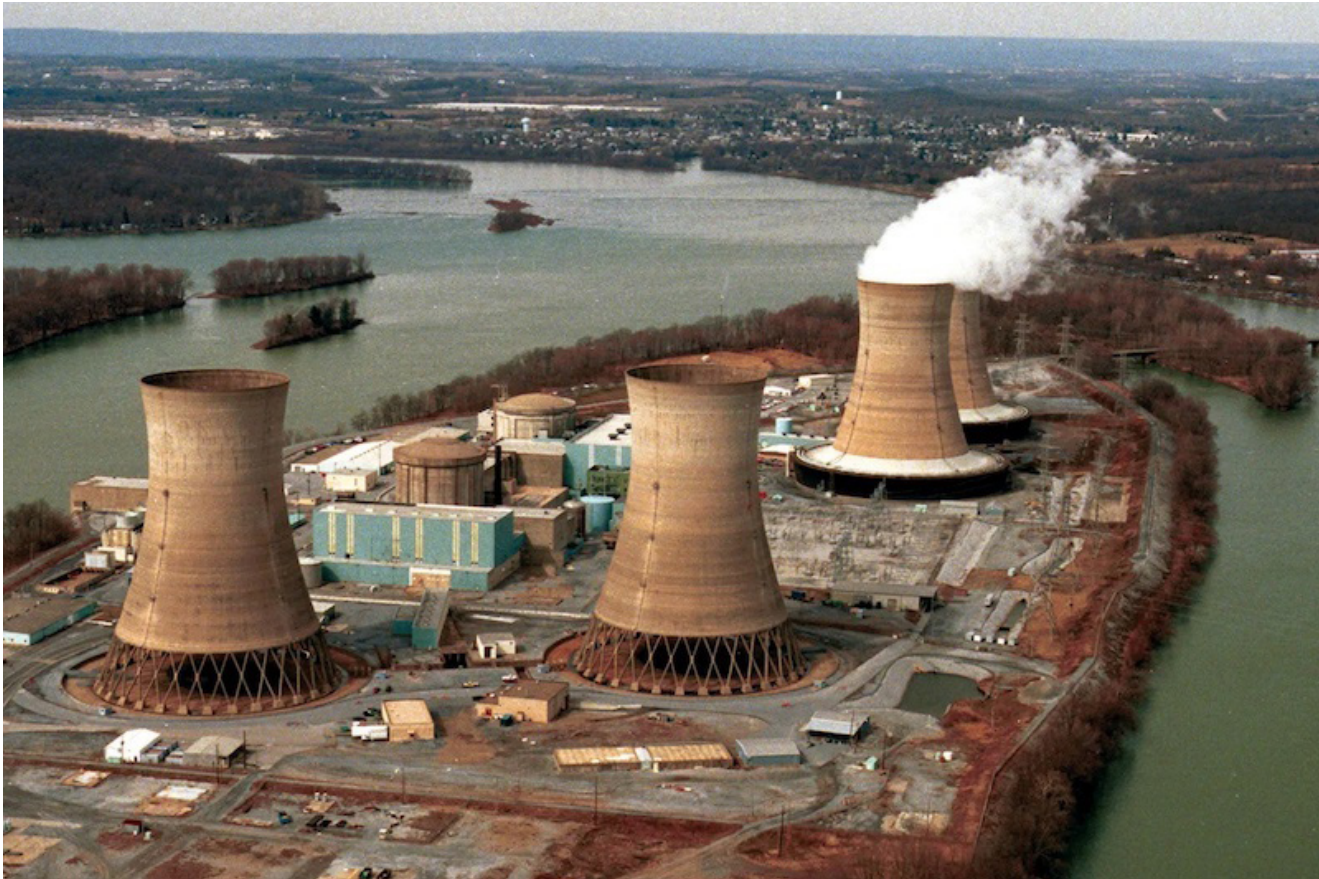
The large round cooling towers of the Three Mile Island nuclear power plant in Pennsylvania became a symbol of the public's fear of nuclear energy after a March 1979 accident at the plant.
