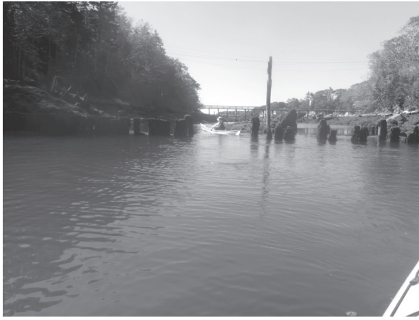
A paddler finds a route through ancient pilings on the inside of Birch Island
