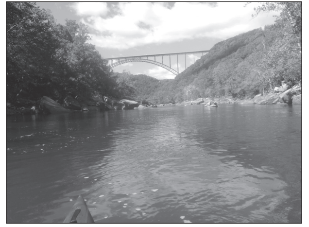
Paddlers approach the New River Bridge
