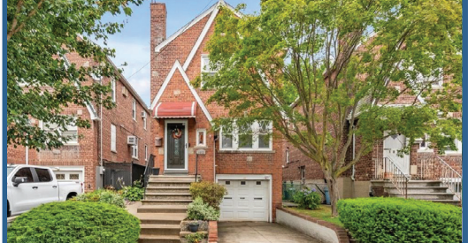
1852 Hering Ave Bronx, NY 10461. Gorgeous Indian Village Tudor 3BR/2Baths. Vincent Buccieri, Lic. Assoc. RE Broker. 917.440.2122
