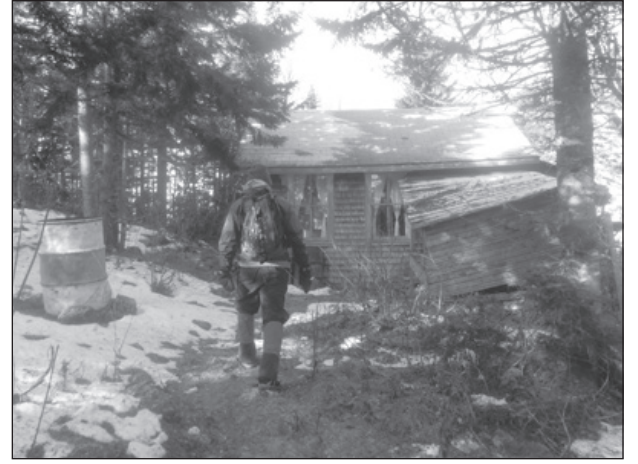
A dilapidated Fire Warden's cabin is located a short distance below the summit
