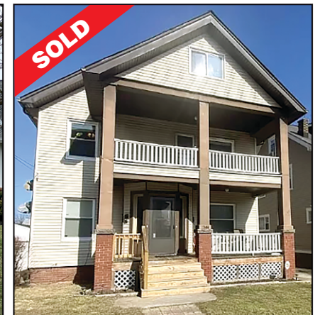
17444 Northwood Ave, Lakewood
