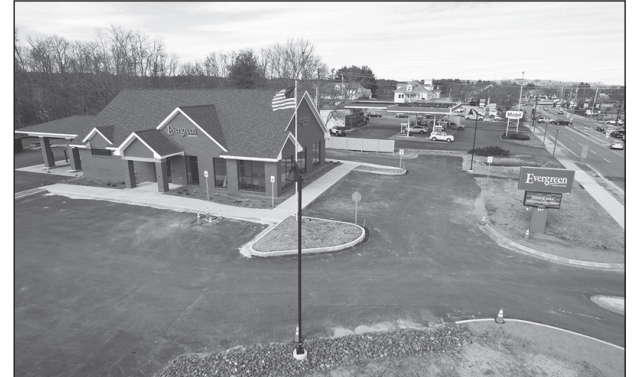
Evergreen CU's Scarborough branch, scheduled to open Saturday, April 20, 2024.
