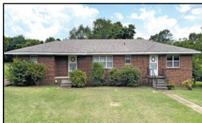
Commercial Potential - 675 Cox Creek Pkwy
