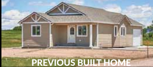
PREVIOUS BUILT HOME
